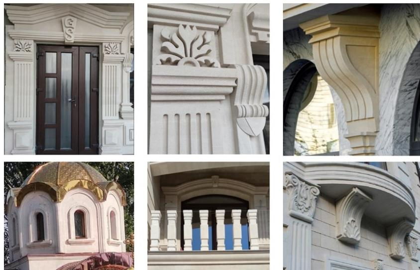
**Figure 5.** Limestone decoration elements for facade rehabilitation.
