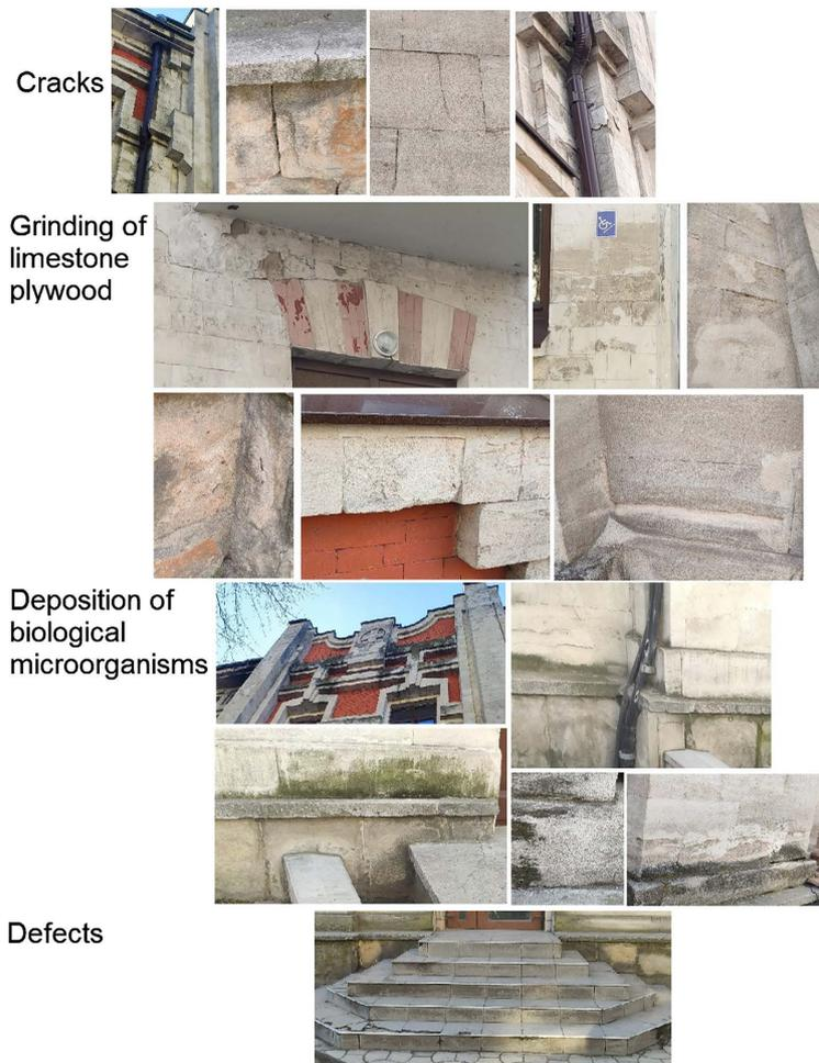
Figure 3. Results of the visual inspection of the building façade.
